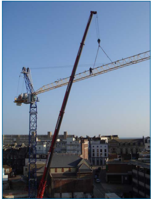
The crane being assembled
